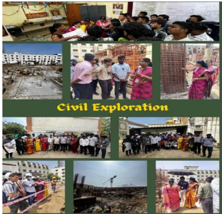
SLMCH Construction site, Adayalampattu Chennai
